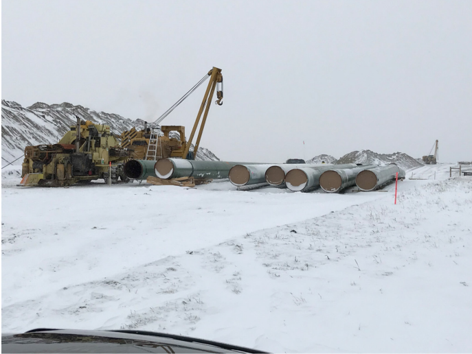
9. Bending crew – km 114+350 – Nov 3, 2017
