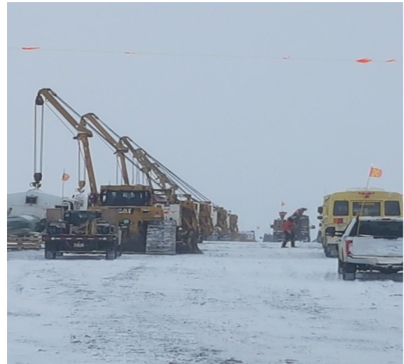
8. Welding activities - km107+800 – Nov 3, 2017
