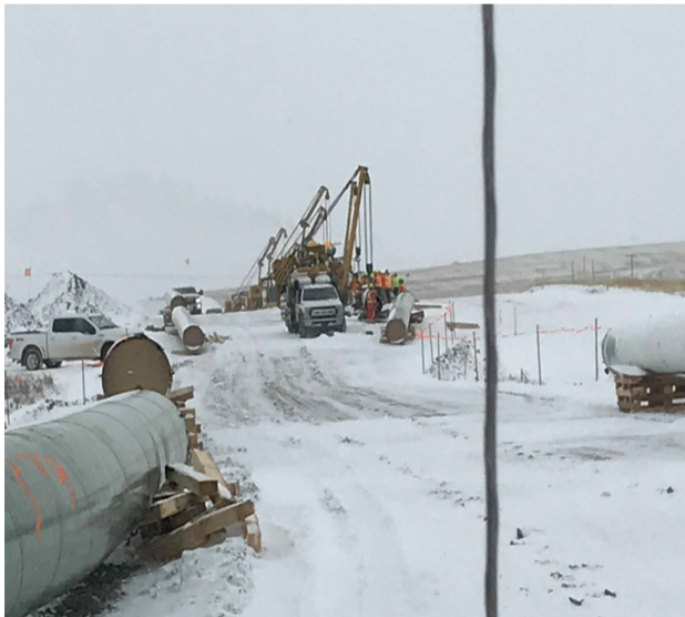
7. Welding crew – km 108+300 – Nov 3, 2017
